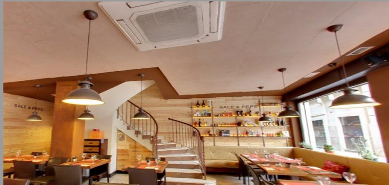
Acoustic Panels on ceiling.
